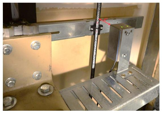
Figure 2-12: APS Camera Mounted 4 Inches From Encoded Tape
