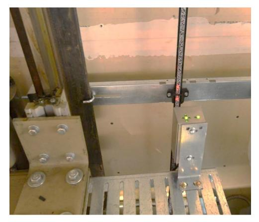
Figure 2-20: APS Selector Alignment Spotlights
