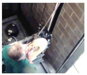
Figure 2-4: Unroll the Encoded Tape
