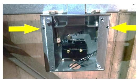
Figure 2-9: Lower Bracket with Springs Properly Compressed to the Marks
