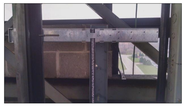
Figure 2-1: Encoded Tape Mounting – Top Bracket
